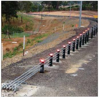
How the FLEXFENCE TL3 End Terminal Works The Flexfence TL3 Terminal is designed to provide a soft gating impact preventing vehicles from launching or snagging. The terminal comprises shortened posts at 1m spacings reducing the angle at which the cables are terminated, thus minimising the potential for vehicle rollover.
