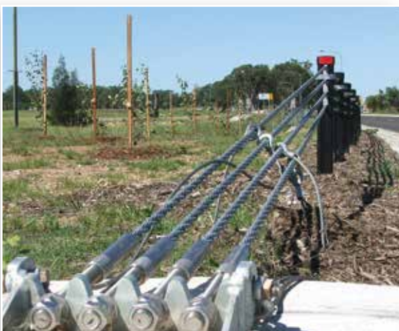
Figure 12: Anchor Block Fitting Arrangement
