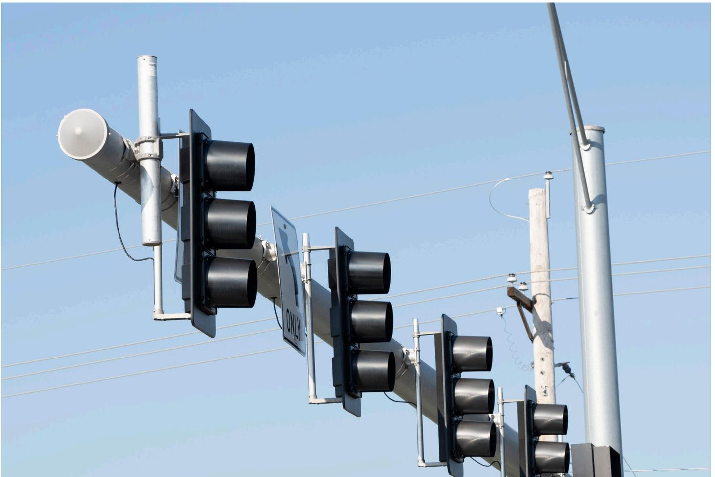
The Valmont Mitigator TR1 Vibration Damper Mounted to a Traffic Light Pole
