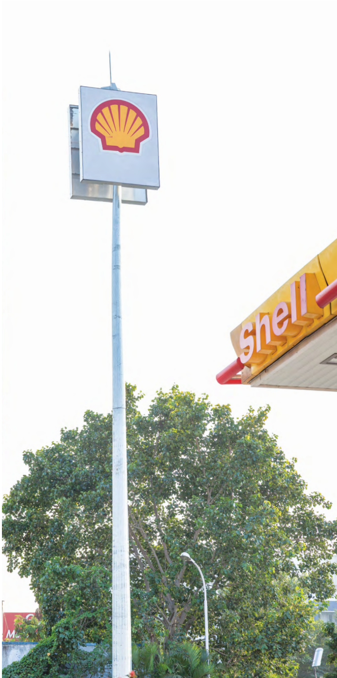
22M SIGNAGE MAST FOR SHELL AT CHENNAI
