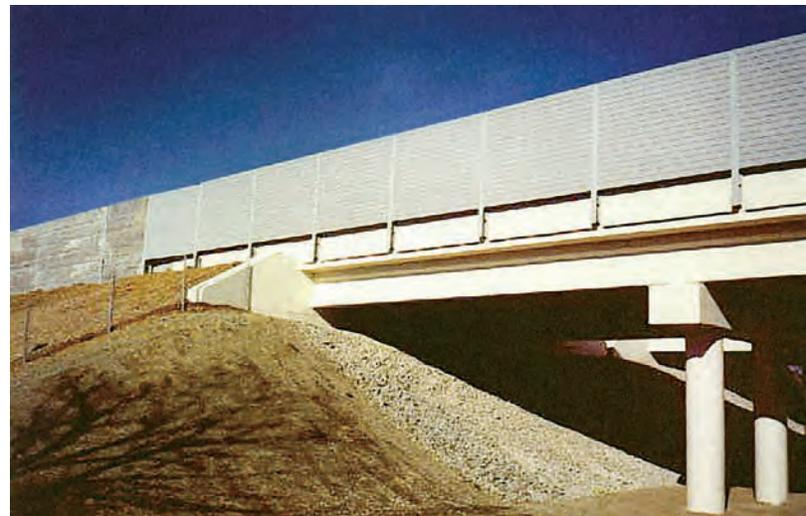
At only 5 to 7 pounds per square foot, AcoustaShield does not add unnecessary weight to bridge structures.
