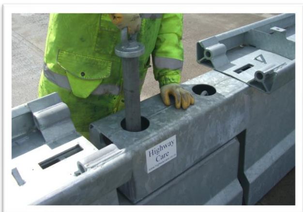
Hinge Pin Being Removed
