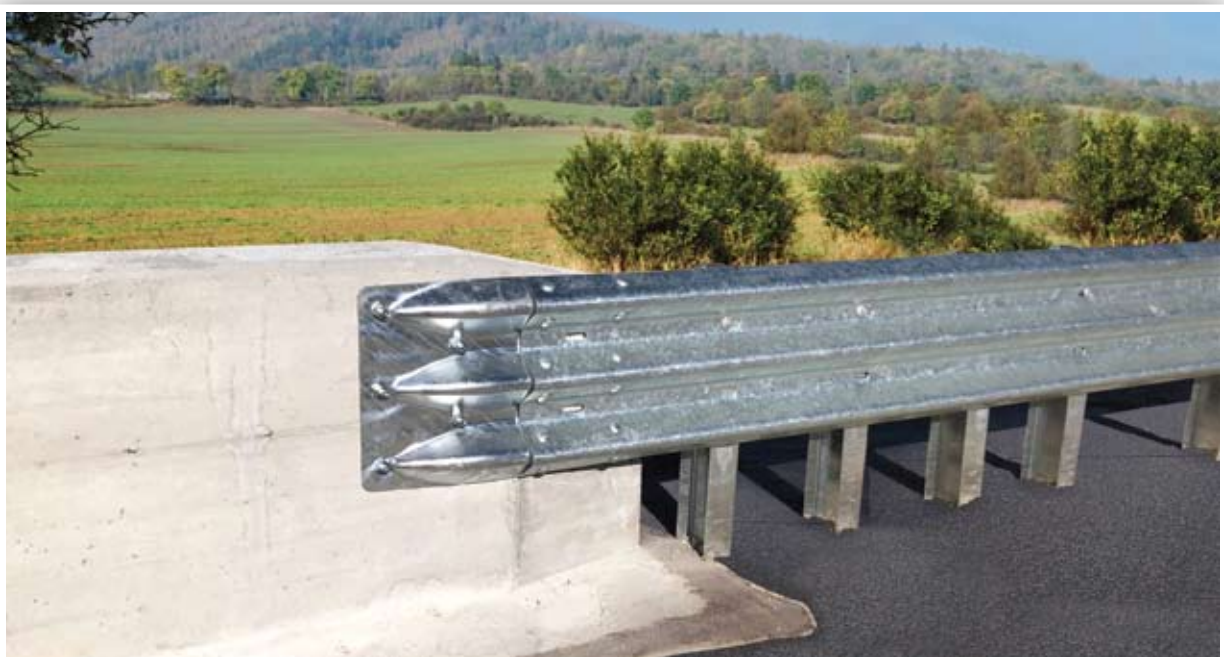
Figure 4: Structural connector to concrete
