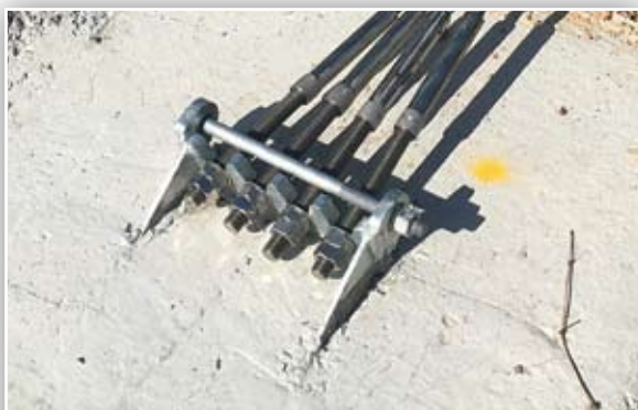
Figure 18: Anchor bracket with locking bolt
