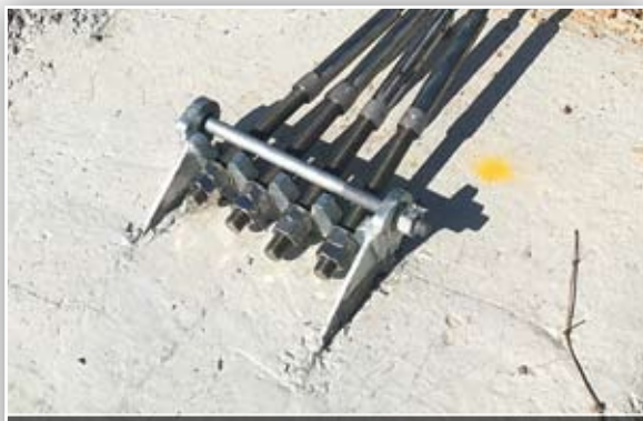
Figure 18: Anchor bracket with locking bolt
