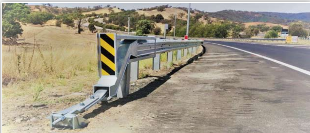
Figure 7: ET-SS End Terminal
