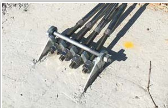
Figure 18: Anchor bracket with locking bolt
