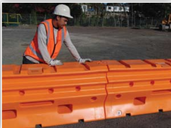
Figure 4: Units are pushed together to align the vertical holes
