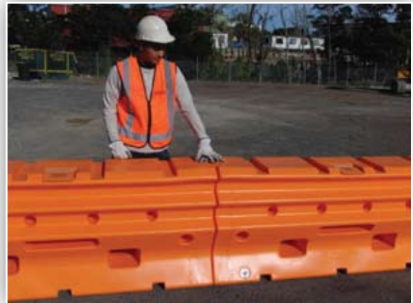
Figure 7: Check the steel pin has gone through the alignment holes.
