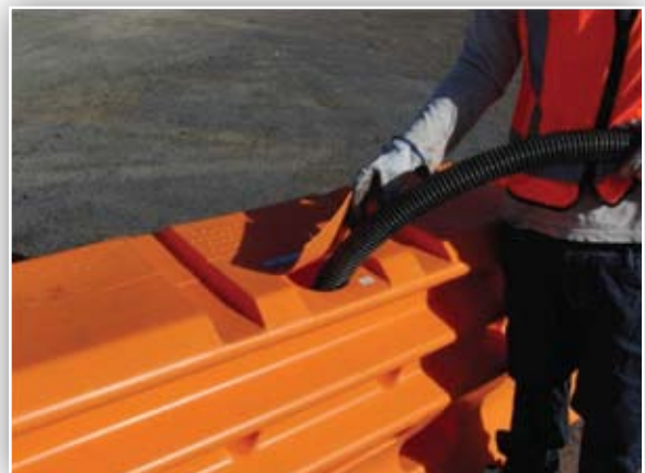
Figure 9: Using a truck mounted tanker fill each unit to the top with water.
