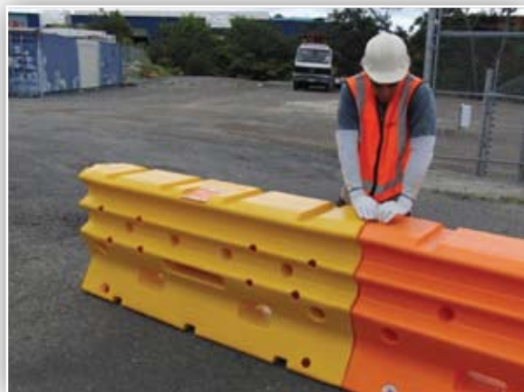
Figure 13: Ensure the steel pin has gone through the alignment holes.
