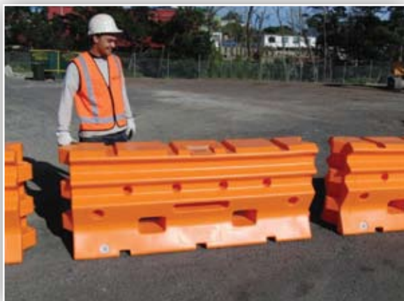
Figure 2: When setting out, ensure the configuration of the ends will fit together.
