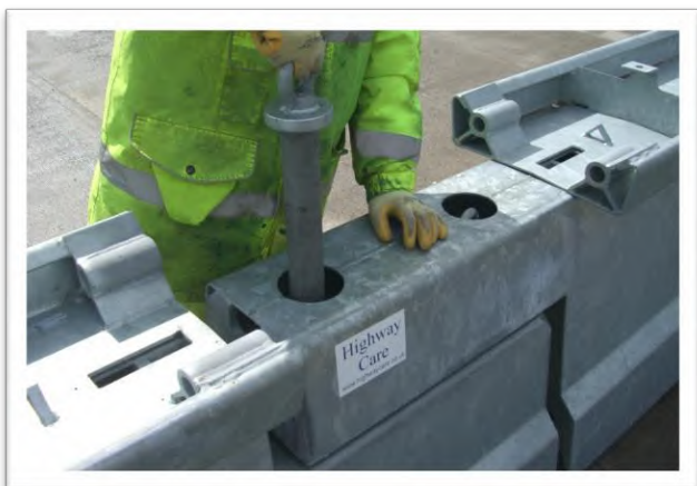
Hinge Pin Being Removed
