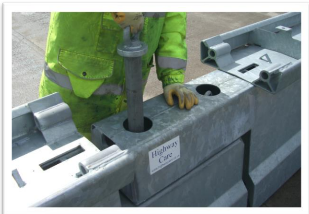
Hinge Pin Being Removed
