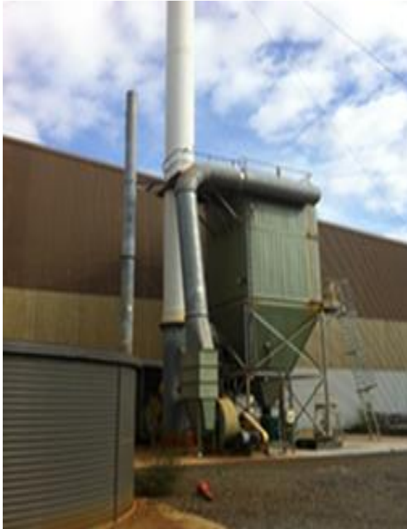
Figure 1 – EPA 1 – Baghouse Stack
