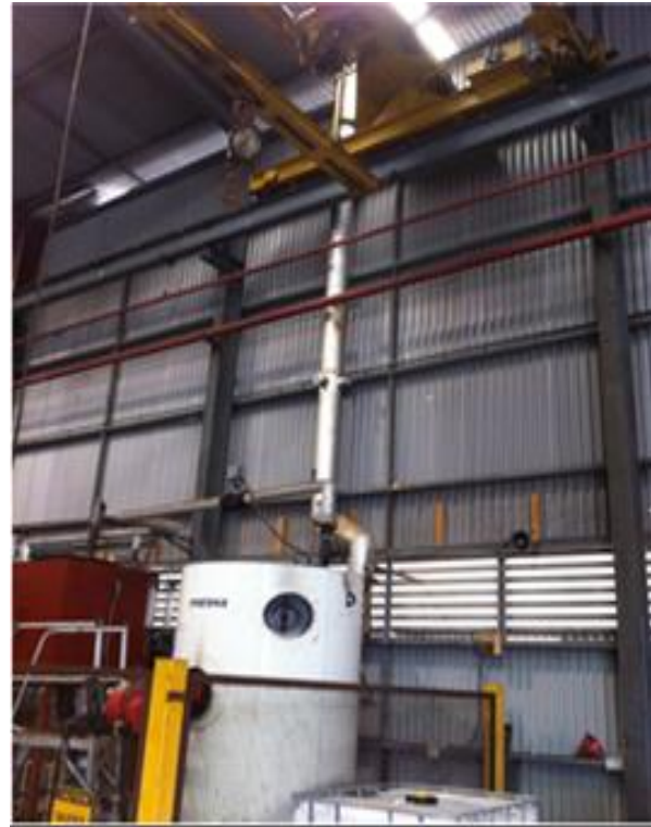
Figure 2 – EPA 2 – Galvanising Area Boiler
