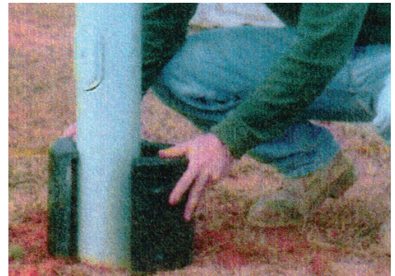
2. Place Pole Guard halves around pole
