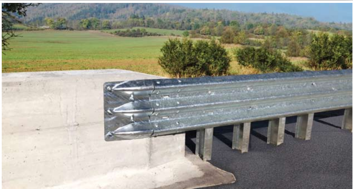
Figure 4: Structural connector to concrete
