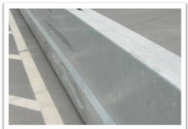
Typical Impact Damage
