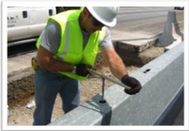
Security Nut Installation
