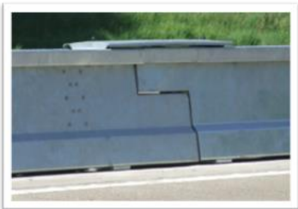
Gate Post & Hinge Joint
