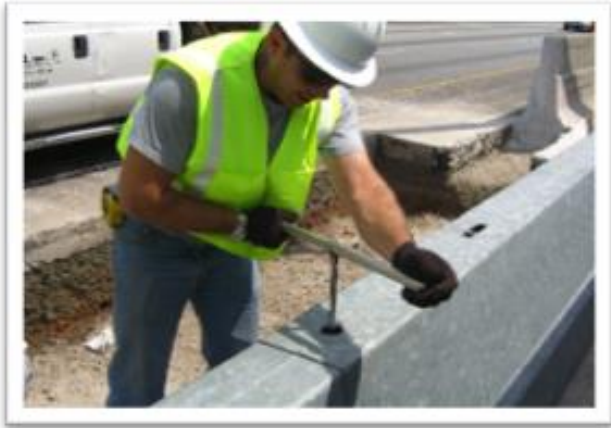
Security Nut Installation
