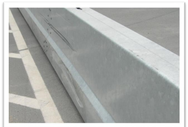
Typical Impact Damage
