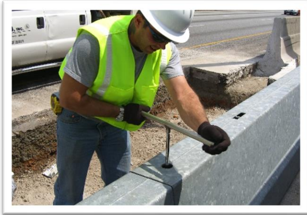
Security Nut Installation
