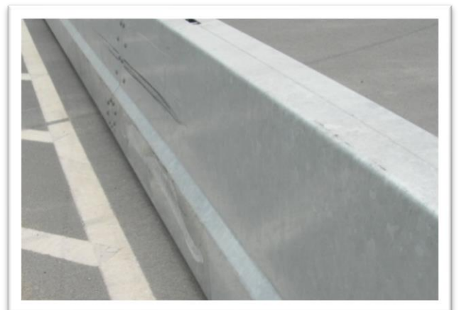
Typical Impact Damage
