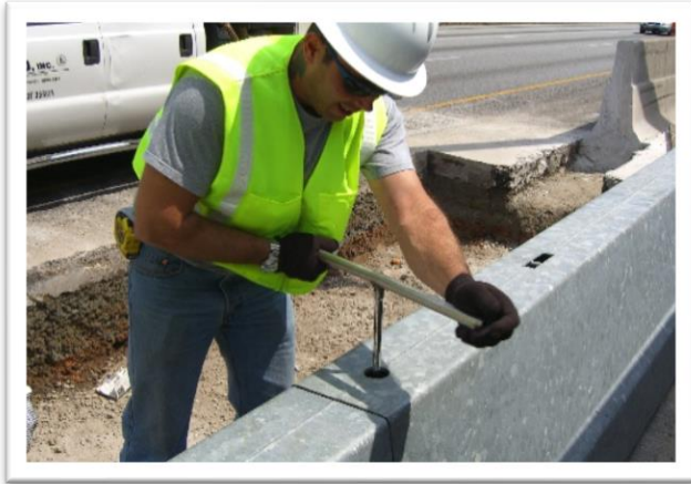
Security Nut Installation
