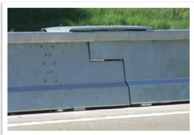
Gate Post & Hinge Joint
