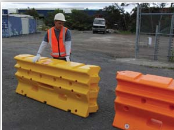
Figure 10: Position the end treatment unit so that the lugs line up with the end barrier unit.
