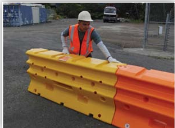
Figure 11: Slide the unit into position so that the vertical holes line up.
