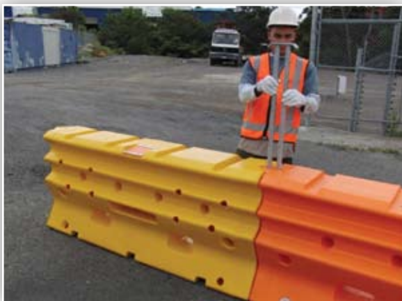
Figure 12: Once the units are aligned, the steel pin can be dropped into the alignment holes.
