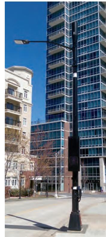
**Valmont structures provides small cell tower and distributed antenna system (das) solutions for outdoor coverage.**
