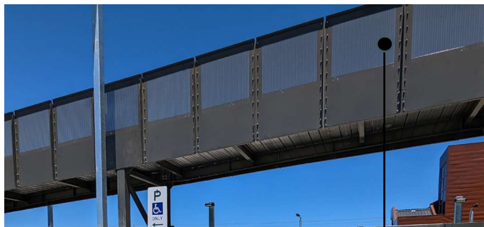
Wairn Ponds, Melbourne Pedestrian Access Footbridge
