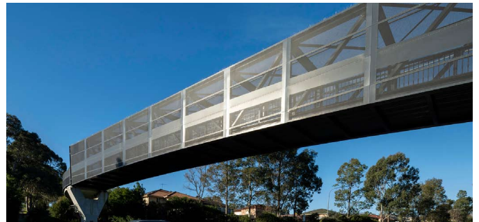
Kingsthorpe, Queensland Pedestrian Bridge Overpass
