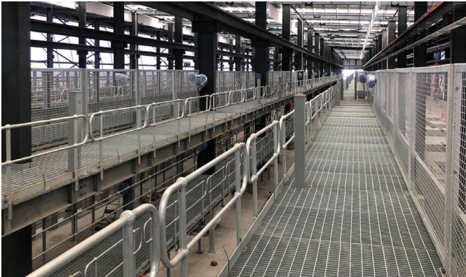
Kangy Angy Rail Maintenance Facility NSW
