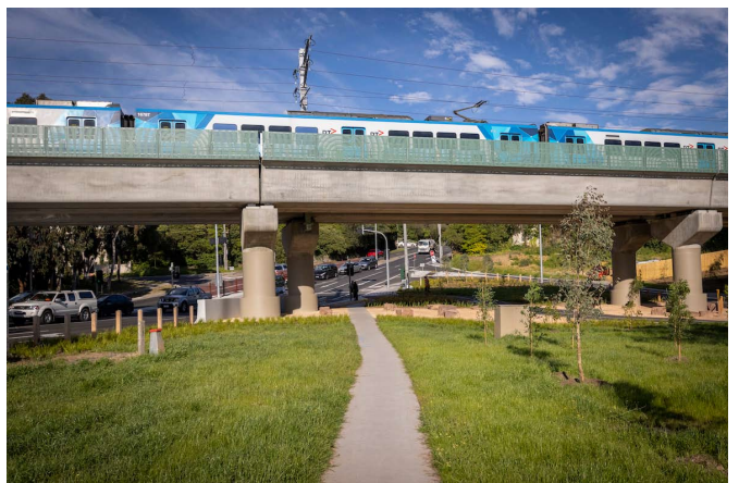
Level Cross - Rail over Road
