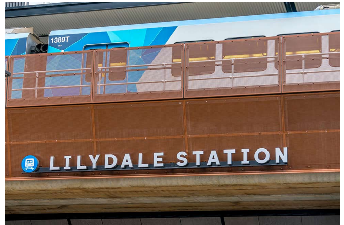
Level Cross - Rail over Road
