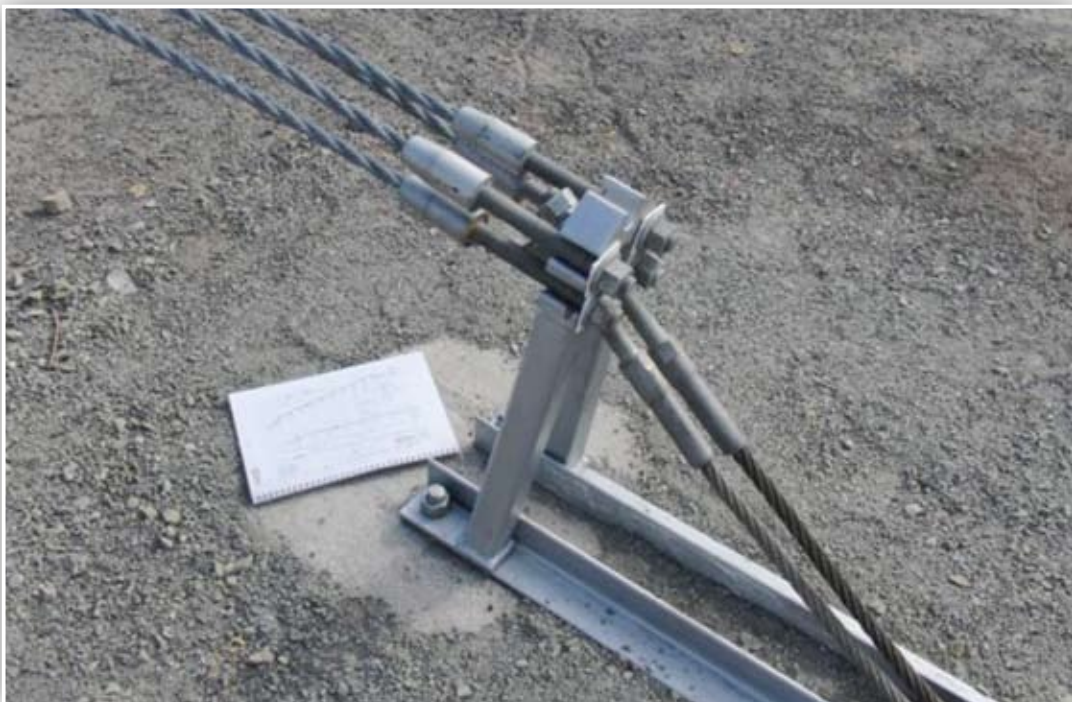
Universal A.T.E. connected to a 4 cable barrier*
