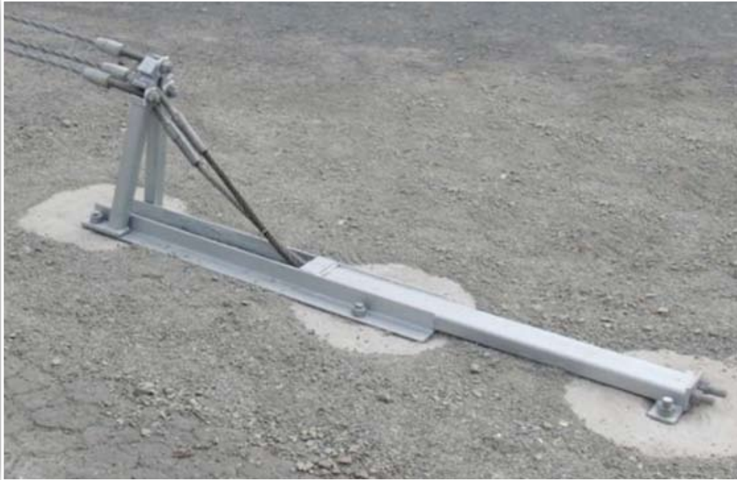
Universal A.T.E. connected to a 3 cable barrier*
