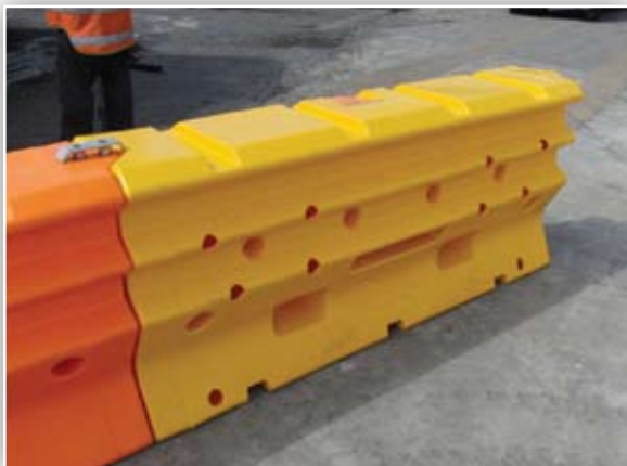
Installed End Treatment
