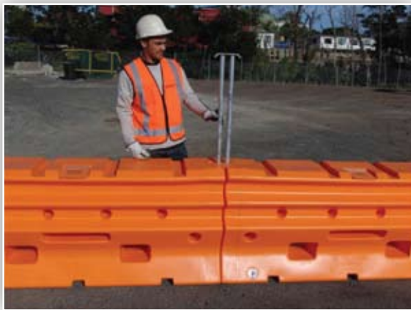
Figure 7: Once the units are aligned, the steel pin can be dropped into the alignment holes.
