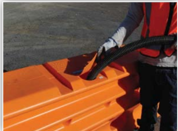
Figure 10: Using a truck mounted tanker fill each unit to the top with water.
