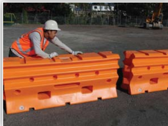
Figure 4: Sliding the units into position.
