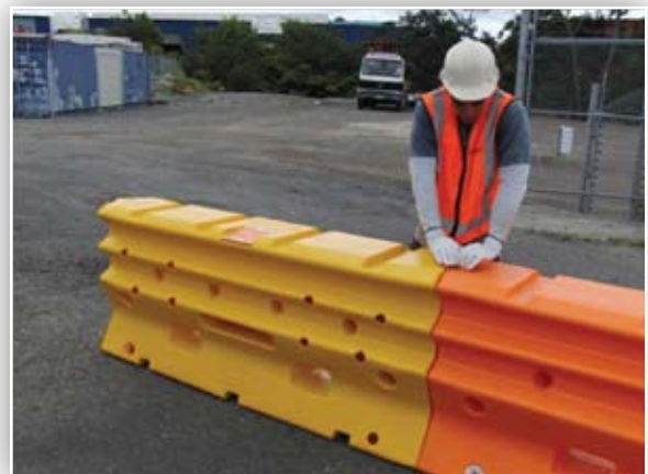
Figure 14: Ensure the steel pin has gone through the alignment holes.
