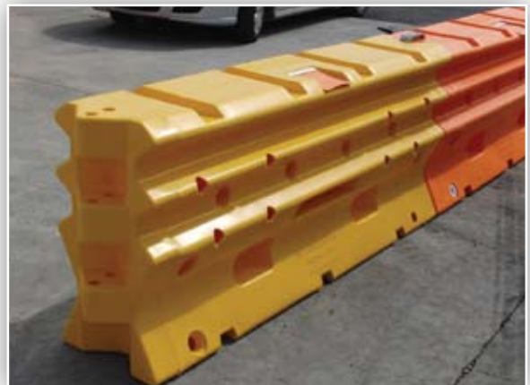
Installed End Treatment
